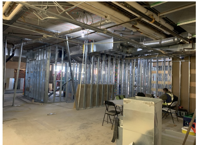
Interior Framing underway
