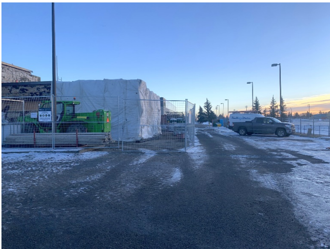
New Exterior Stairs - hoarding
