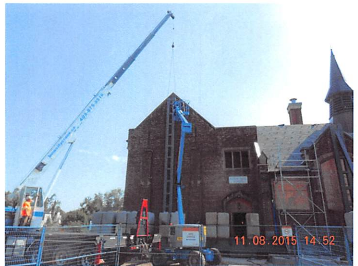
Steel façade retention frame being positioned →
