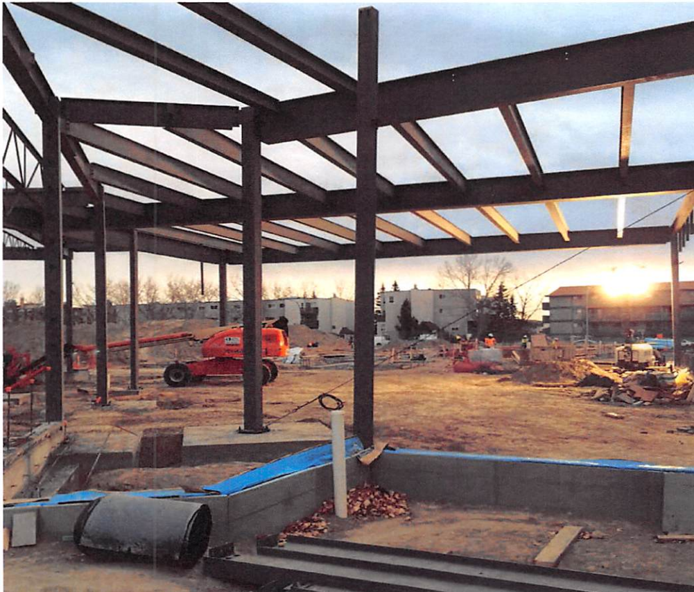
Structural Steel Erection in the Common Space (centre) of the building, looking East
