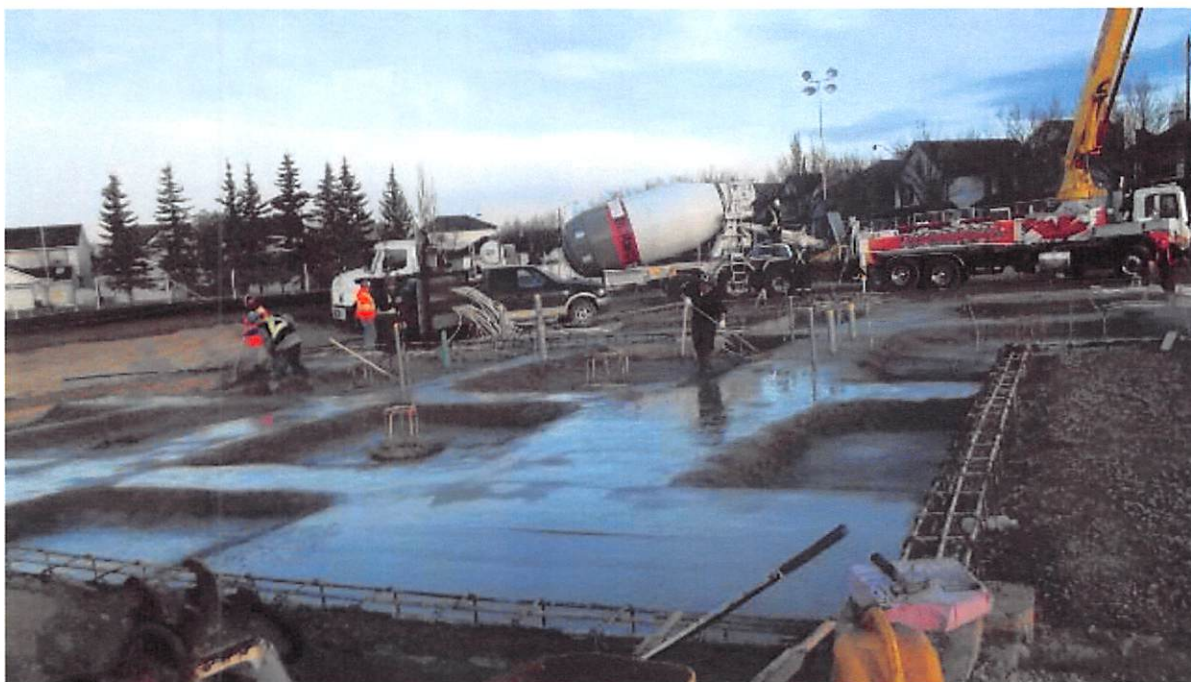
Mud-slab placing October 29, 2015
