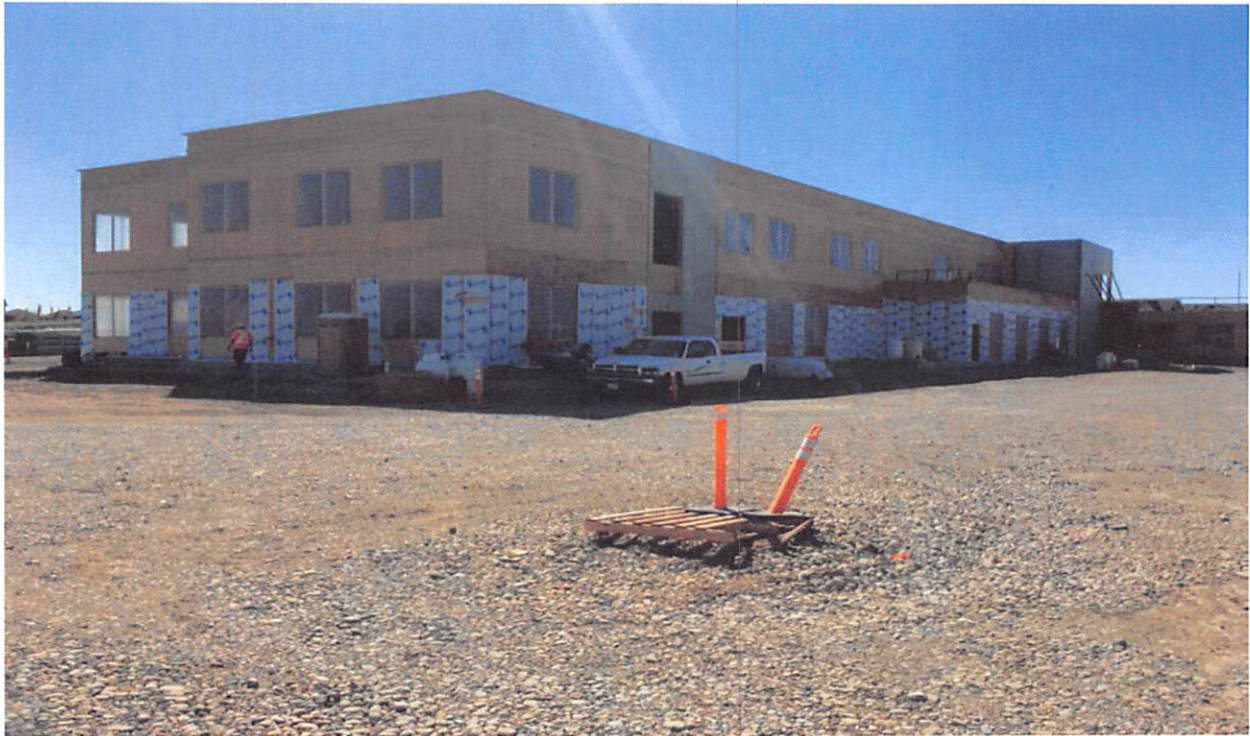
Building 2 Elevation, moisture barrier started
