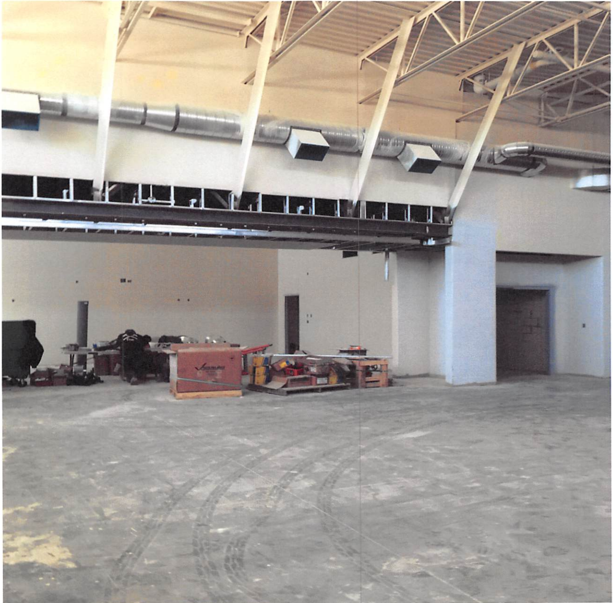
Clerestory ceiling painting, Horizontal HVAC and moveable wall support structure
