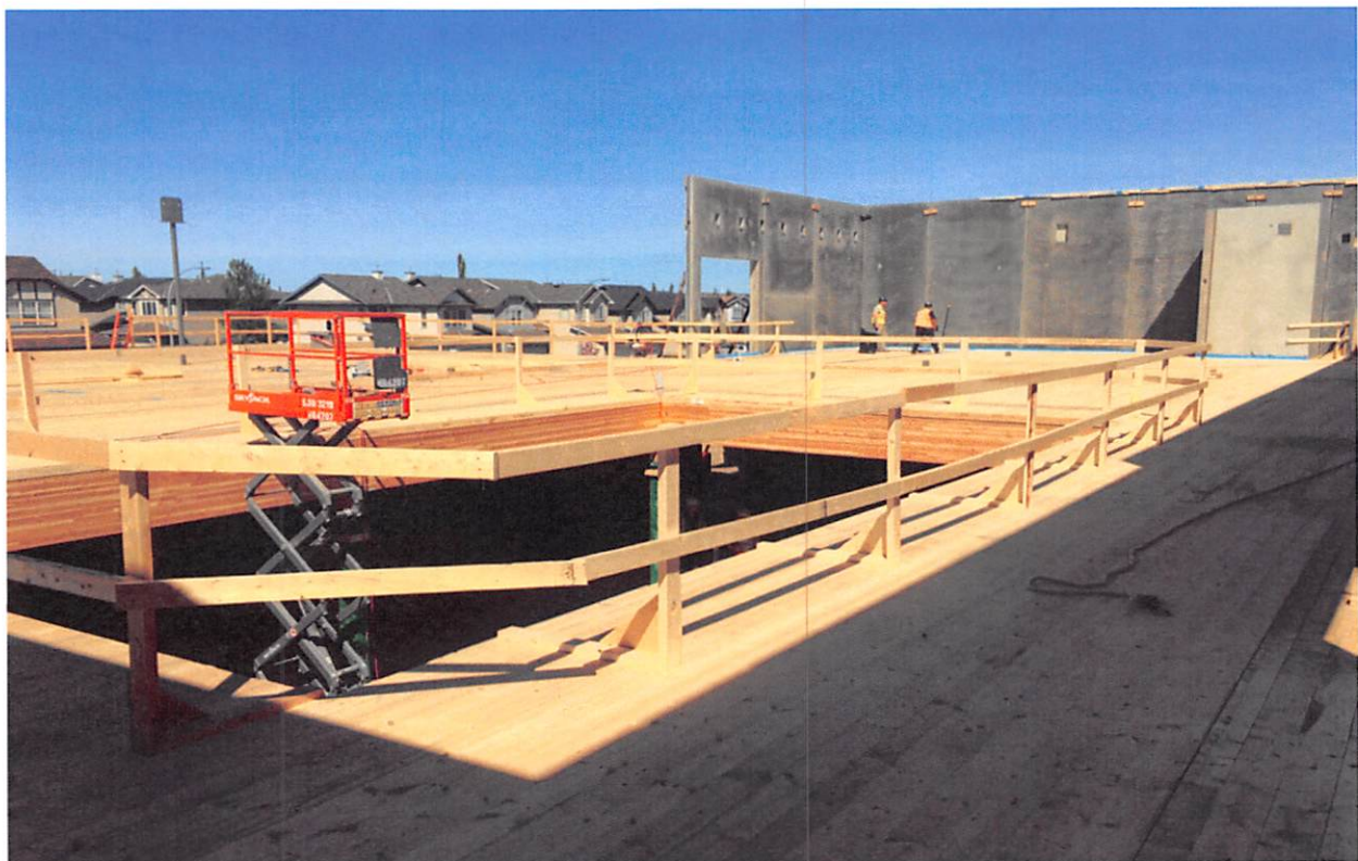
CLT and Precast Panel Installation – Building 1
