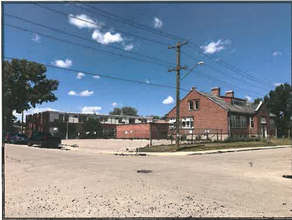
4. VIEW OF THE SUBJECT PROPERTY LOOKING TO THE NORTHWEST
