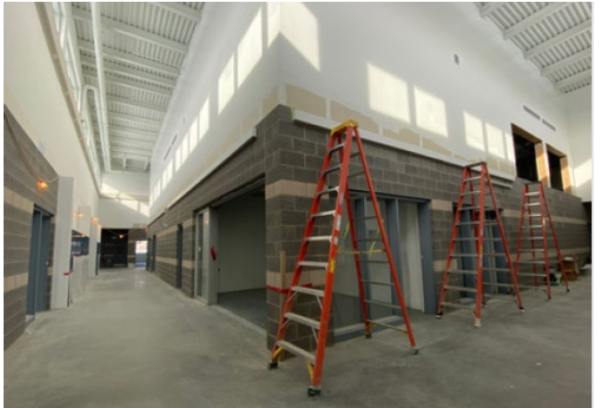
2nd Floor hallway – classroom wing
