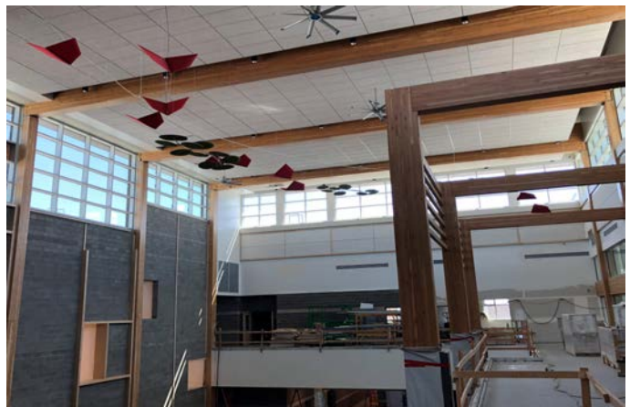
Main Gathering Space - Ceiling
