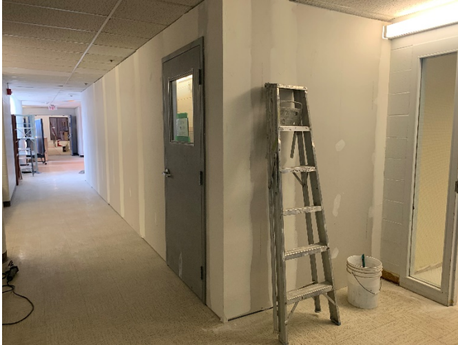
Hoarding – 2 nd Floor
