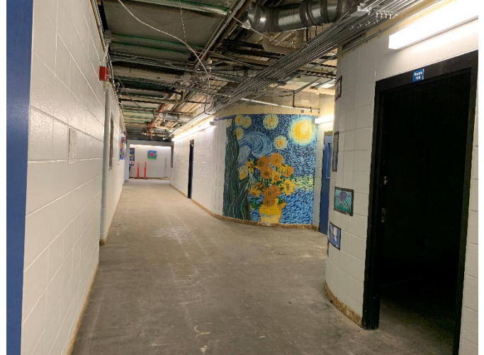
Main Floor Corridor - Demo
