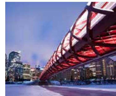
Peace Bridge in Sunnyside
