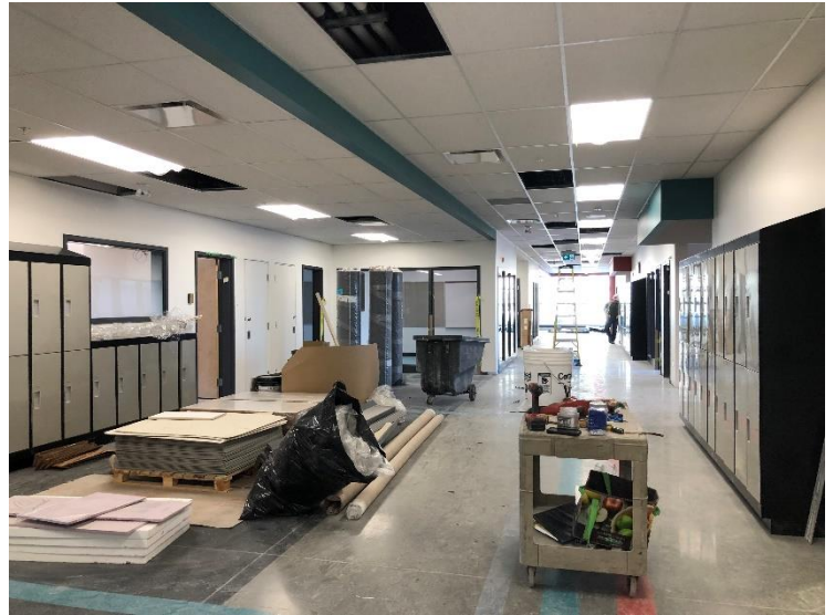
Figure 4: Hallway – Jr. High Section
